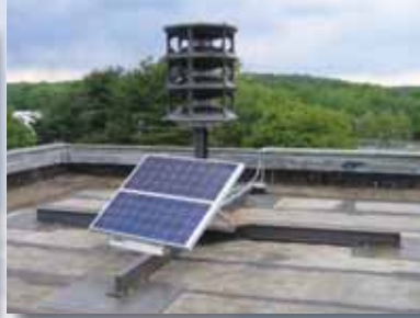
RTM Roof mount and SBC280 solar power options
